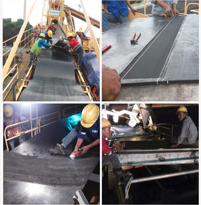
REPLACING AND HOT SPlicing BELT CONVEYOR PT Lestari Banten Energi
