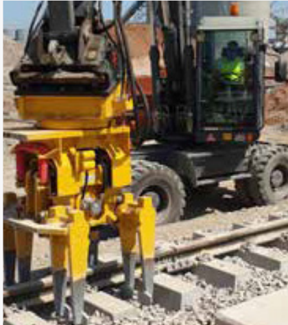
Construction and Renovation
