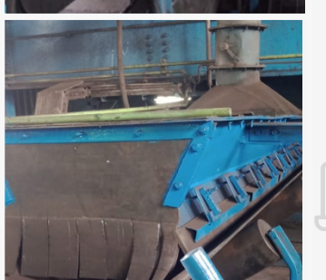
REKONDISI INLET CHUTE BC 702 AB UNIT 7 PT PLN Indonesia Power Suralaya PGU
