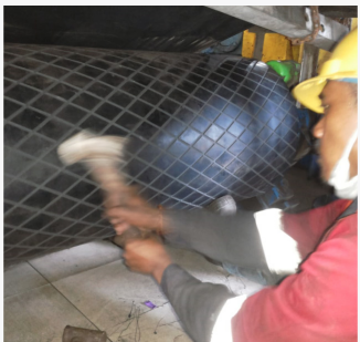
RELAGGING PULLEY DAN SPLICING BELT CONVEYOR PT Lestari Banten Energi
