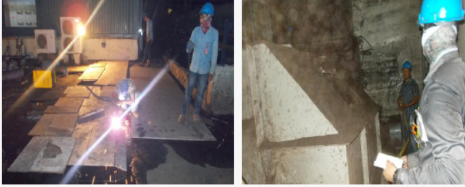
CHUTE REPAIR SERVICES PT PLN Indonesia Power UBP Suralaya Unit 1-7
