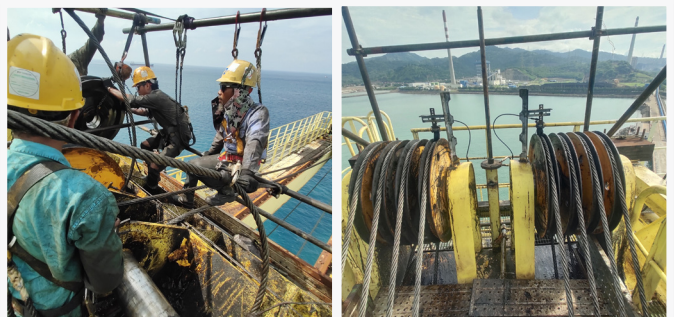
SHEAVES PULLEY REPLACEMENT AND REPOSITION AT SHIP UNLOADER PT Lestari Banten Energi
